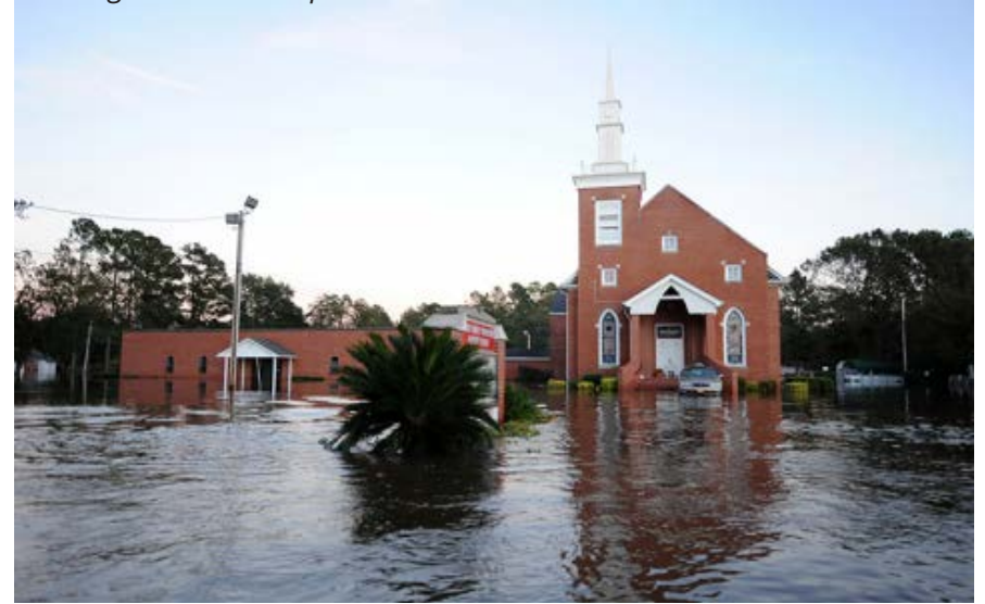
Flooding in Lumberton post Hurricane Matthew
