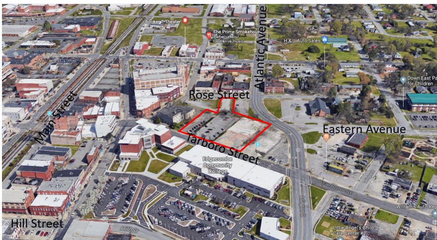
Aerial view of Tarboro Street Site
